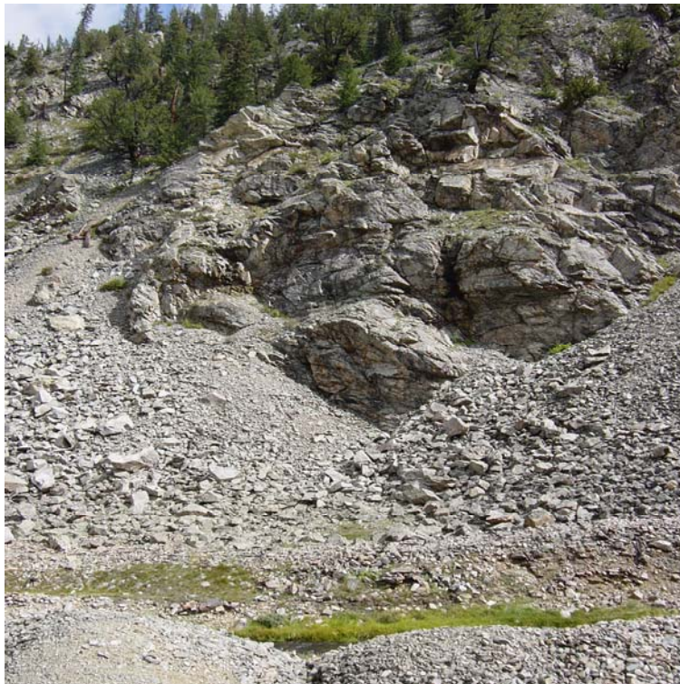
Photo 2.2 Recent rock fall material
